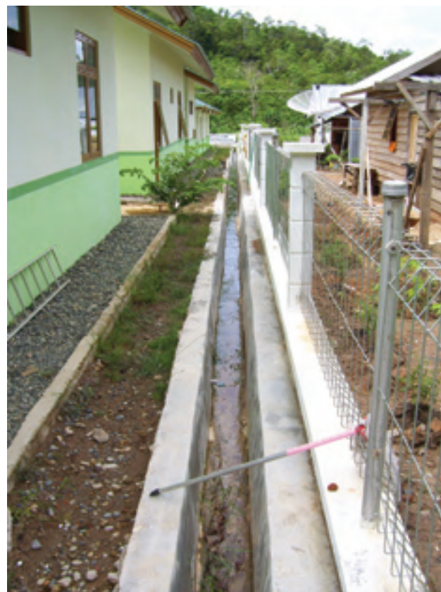
SITE DRAINAGE REDUCED VULNERABILITY TO FLOODING
