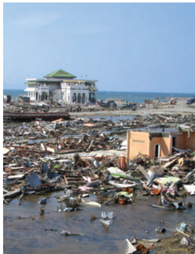
DAMAGE IN BANDA ACEH
