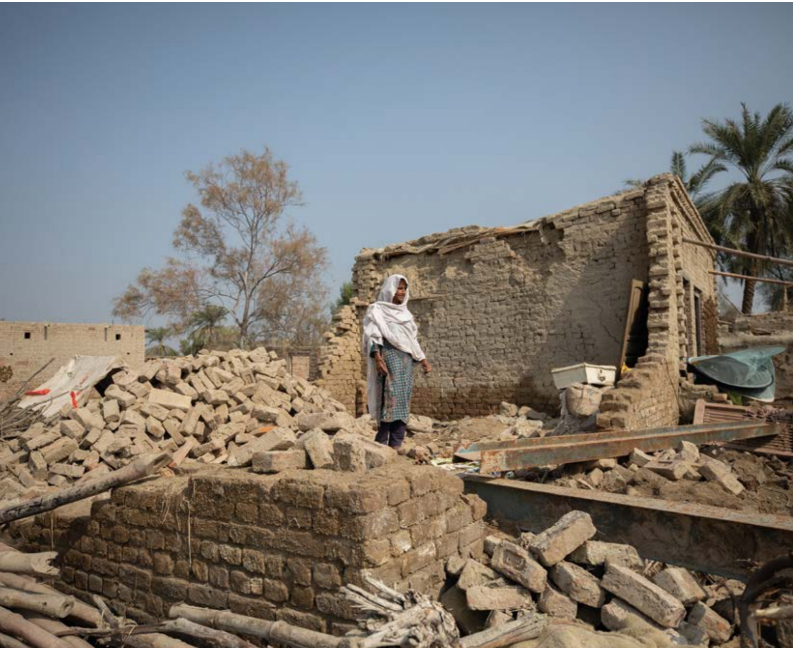
Standing where her house once stood, 35 year old widow, Noor Khatoon gave birth to a baby girl two months ago right after her husband died when the roof of their house collapsed on him. © Khaula Jamil
