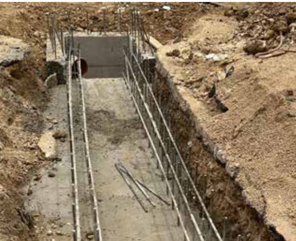
DEC funded rehabilitation work is carried out on a stormwater system to prevent flooding and maintain access to clean water in a conflict-affected area of southern Beirut. © World Vision
