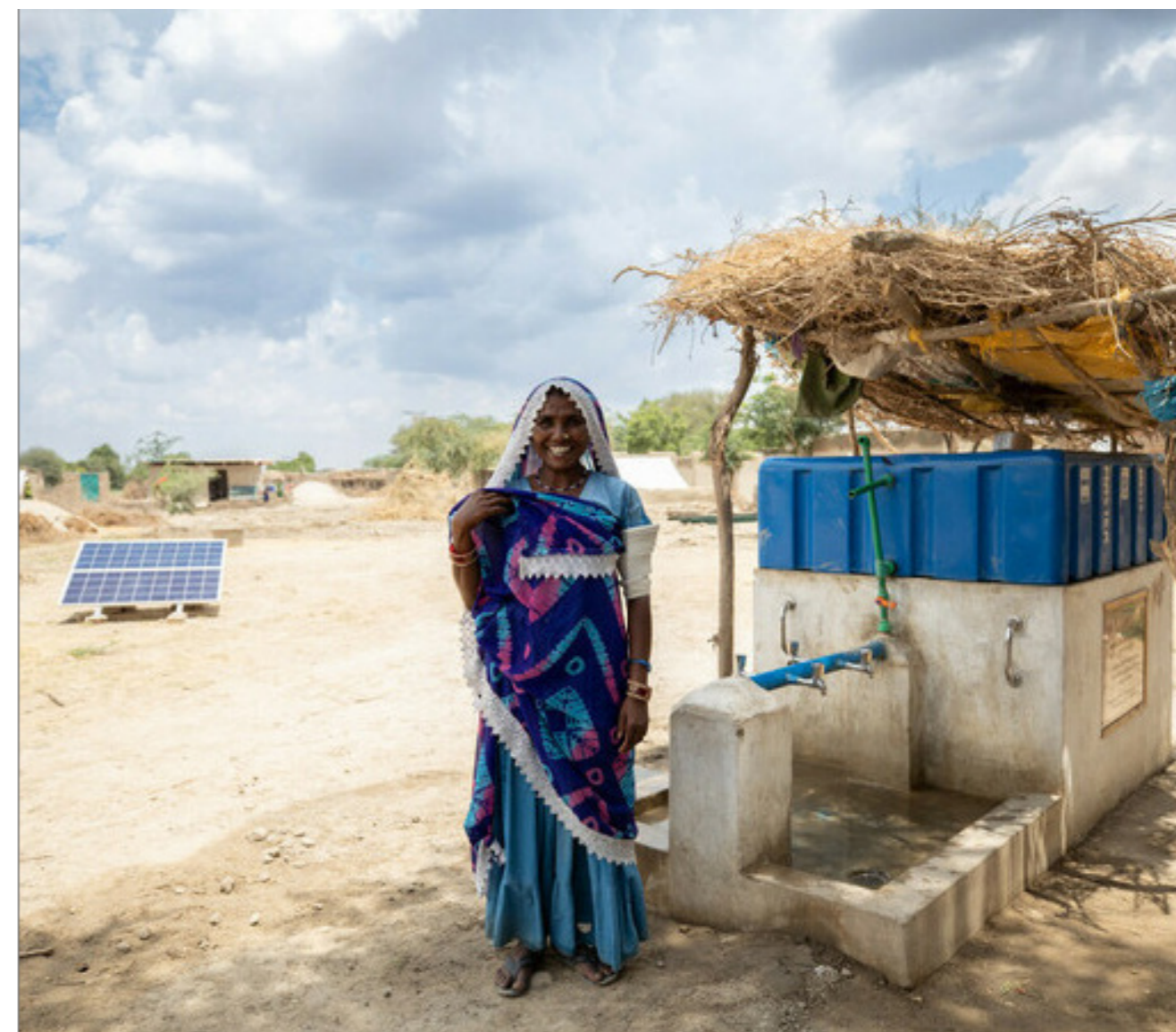
A DEC member and its implementing partners provided a village in Sindh, Pakistan, with a solar water supply system. Photo: © International Rescue Committee
