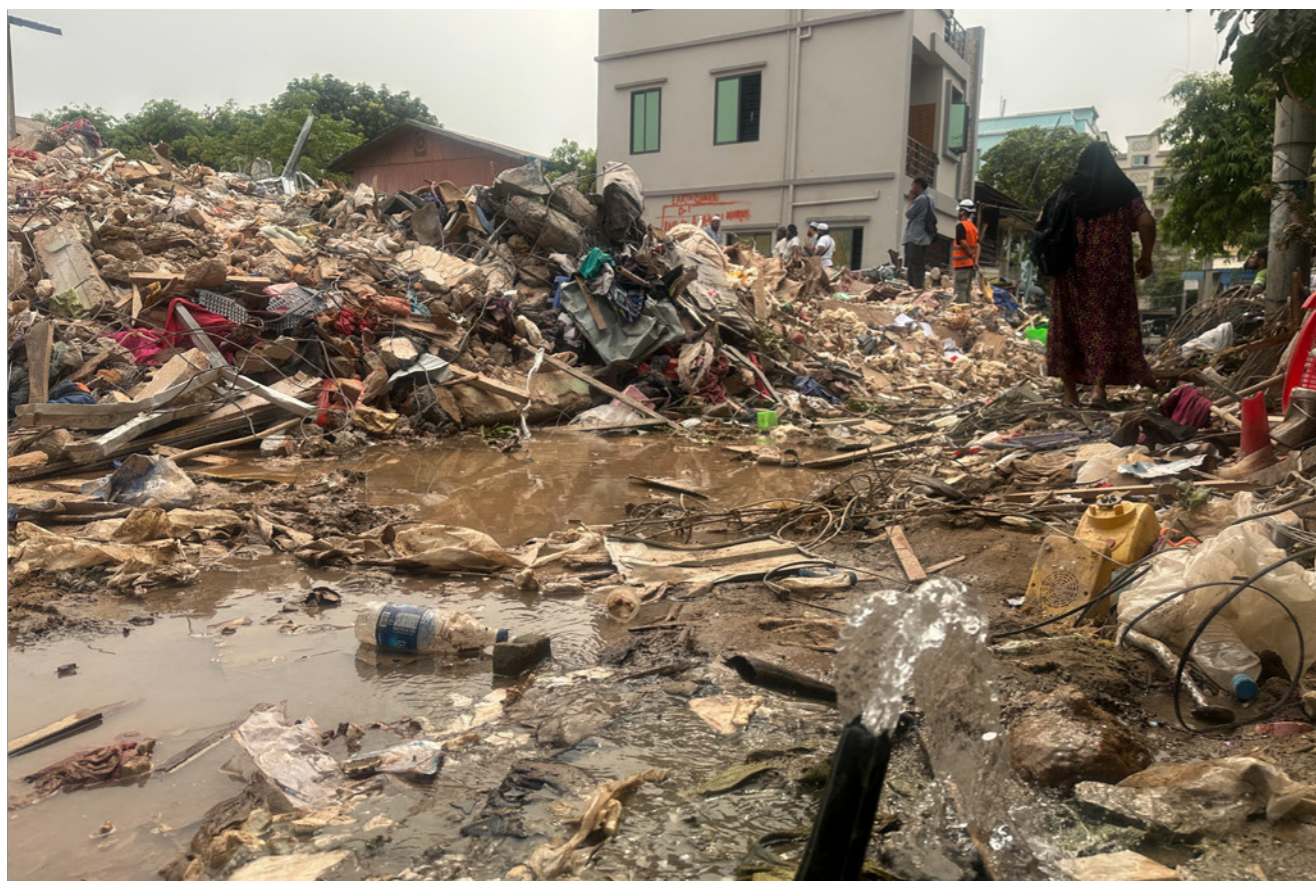
Volunteers work through the rubble of a collapsed apartment building following the recent earthquake in Mandalay, Myanmar Photo: © Arete/DEC
