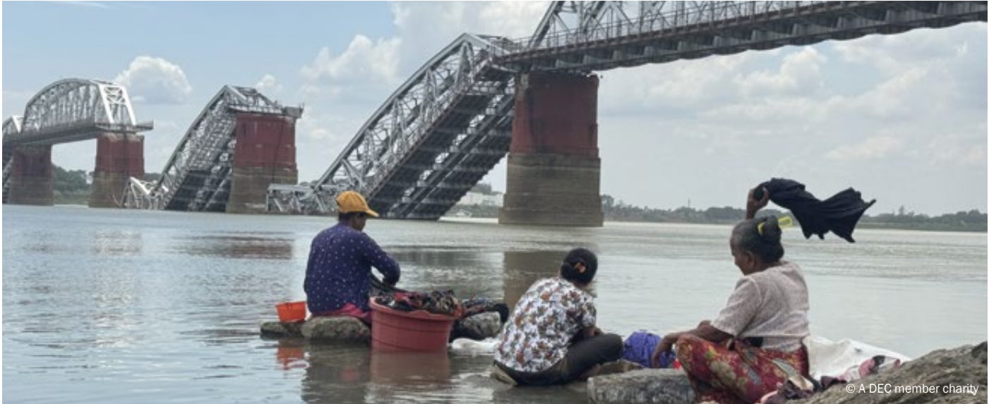
Members of a rural community wash clothes in front of the collapsed Ava Bridge in Sagaing following the earthquake in Myanmar, April 2025. © A DEC member charity
