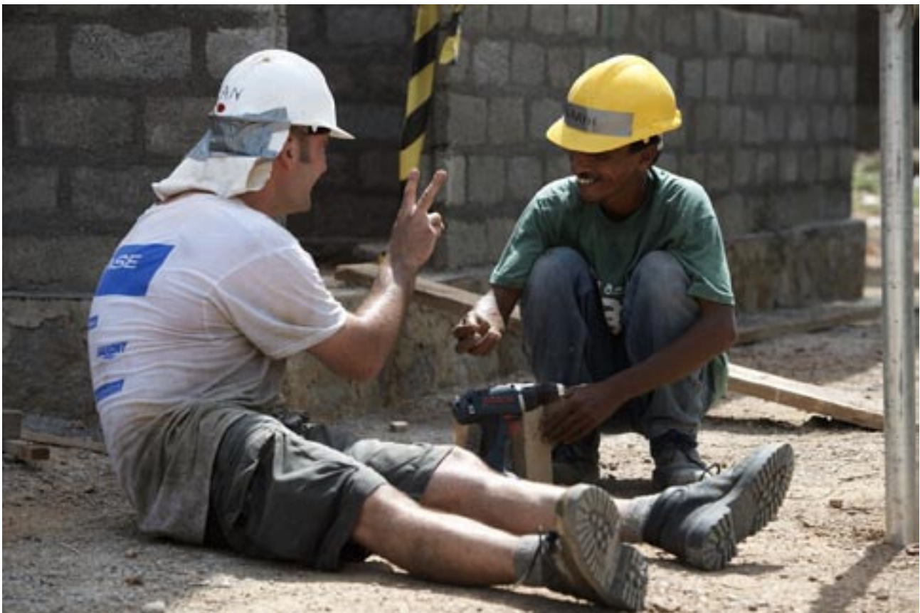
Communicating Across Cultures; Serco Employees working with local staff to rebuild houses in Sri Lanka (Photograph courtesy Barry Willis)
